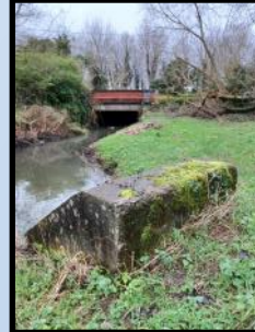
The bridge & brook Sealand Rd
